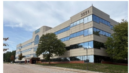
Photo of building at 3551 Hamlin Road
