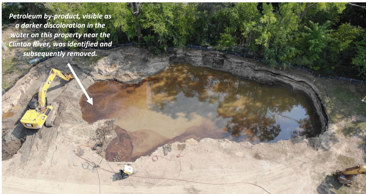
Photo of 3180 Auburn Road taken during the clean-up
