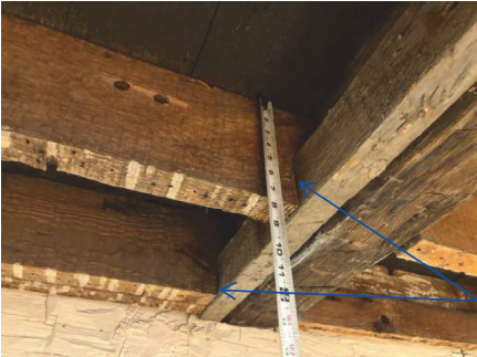
Notched joists above kitchen area. Attic space is currently unused. If planning to use, evaluate reinforcing notched ends
