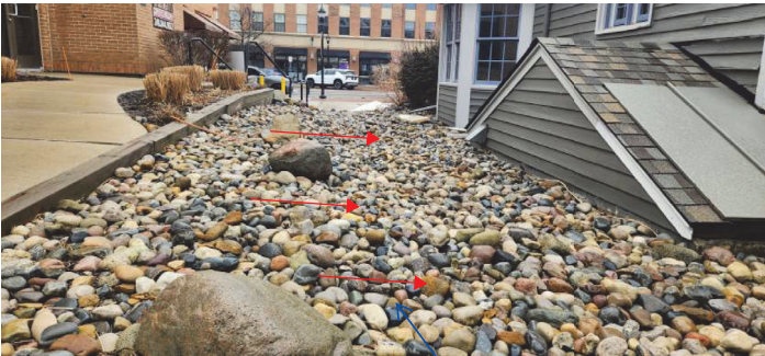
Water leakage into basement after rain event
