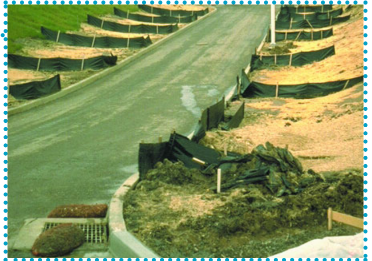
erosion controls at development
