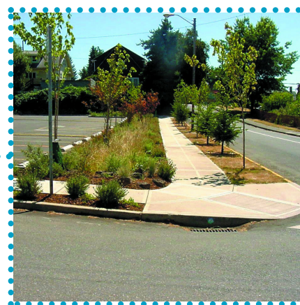
same parking lot with stormwater swales
