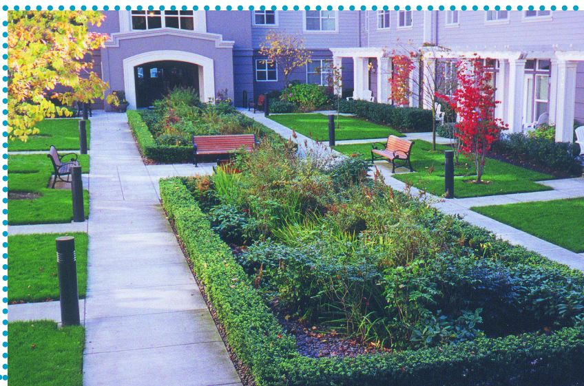
Buckman Heights stormwater planters
