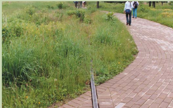
9. level spreader and filter strip at Coffee Creek Center (Chesterton, Indiana)
