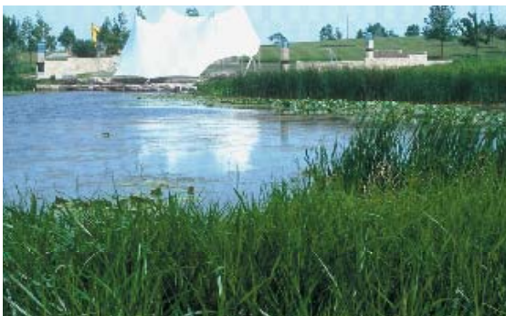
10. naturalized wet detention basin at Sears Prairie Stone (Hoffman Estates, Illinois)
