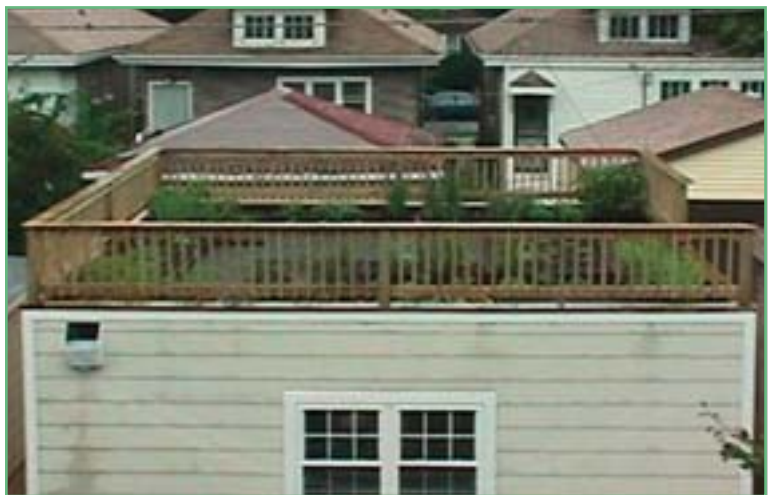
Chicago's Green Bungalows program encourages the use of green roofs. Green roofs are one of the many BMPs that will be recommended in this guide to handle stormwater runoff.
