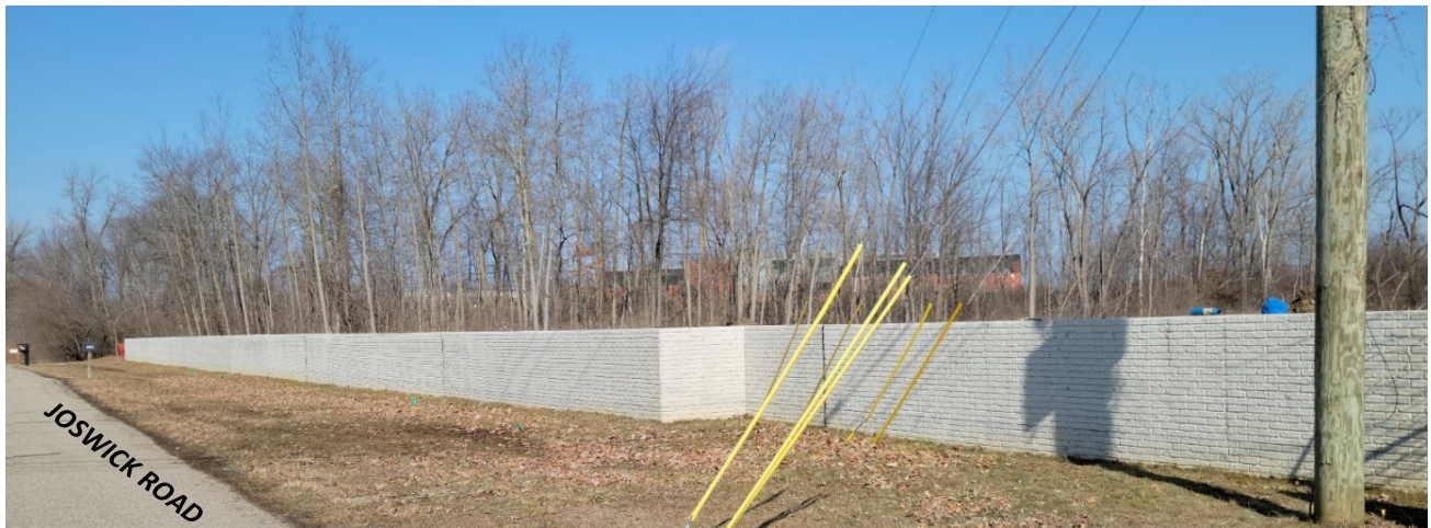
Photo of the new screen wall built in 2021 to match the existing screen wall along Joswick to the south
