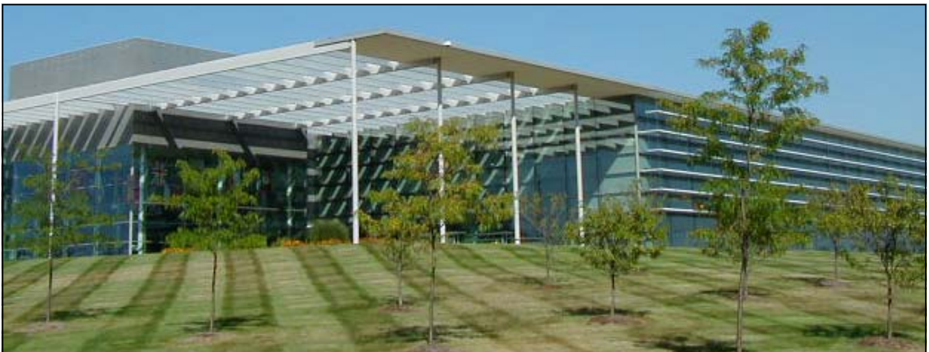
Valeo Building – 4100 N. Atlantic Boulevard
